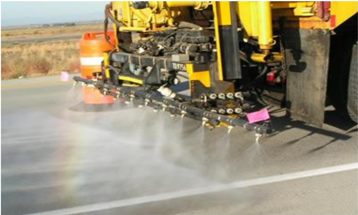
SPRAYING 30% LITHIUM NITRATE SOLUTION ON CONCRETE PAVEMENT NEAR MOUNTAIN HOME
